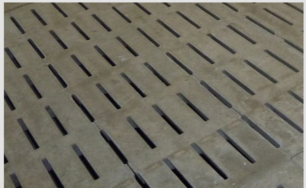
Split tiles with Maleki-SlagSil
