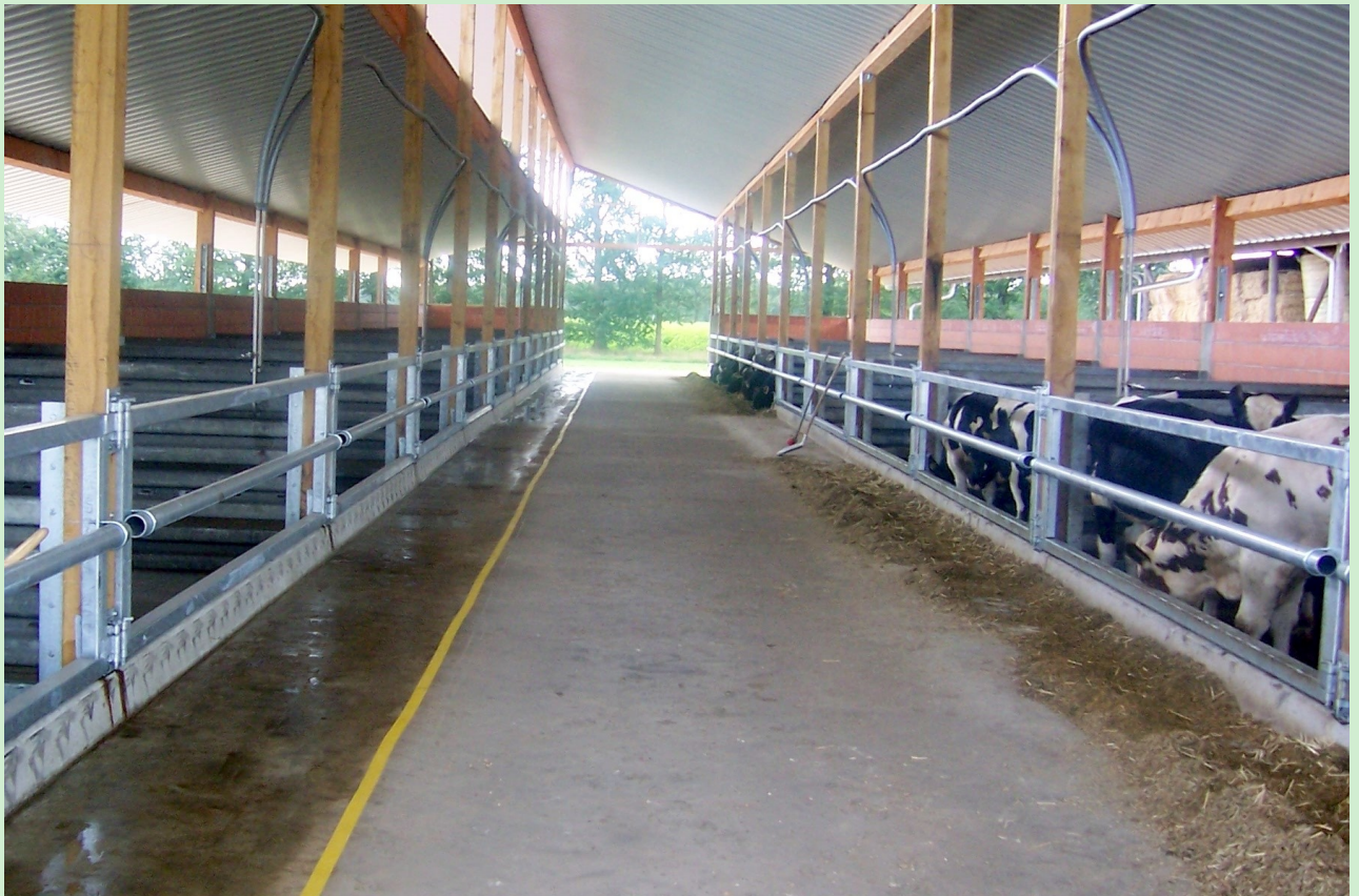
Coating of a feed table with Maleki-DW 100 and Maleki-LL 100 to prevent corrosion damage.
