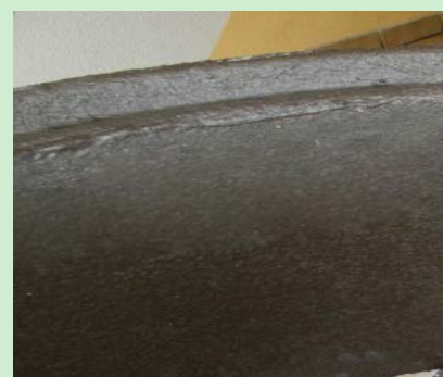
Coating of a tank for silage storage.
