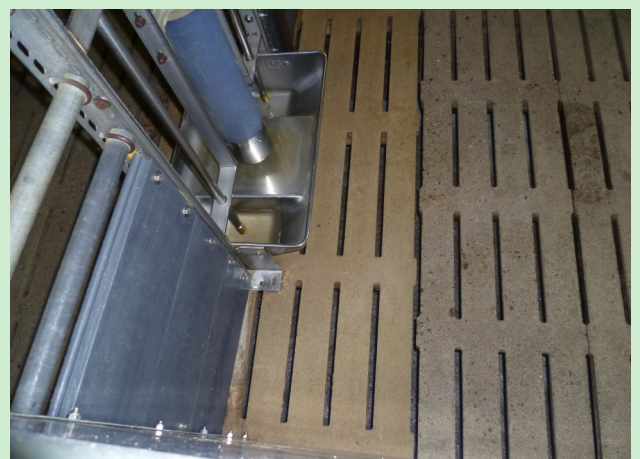
Slatted floor treated with Maleki-DW 100 and Maleki-LL 100 after 2 years of feed acid exposure.
