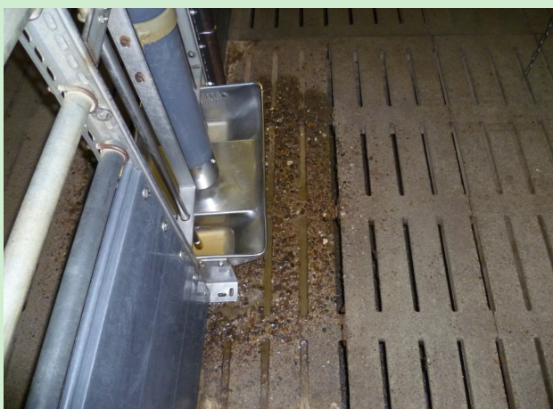
Acid erosion after 2 years of exposure to feed acids.
