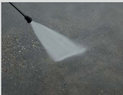
Cleaning by high pressure flushing
