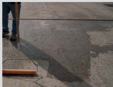
Application with a roller
